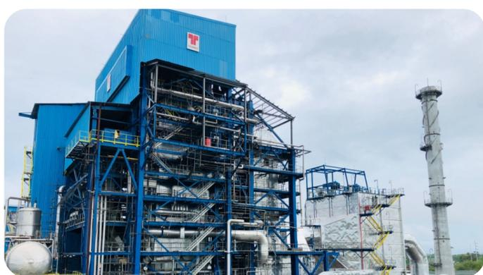
40 MW Boiler Turbine Generator (BTG) supplying steam and power to the sugar and refinery factory
